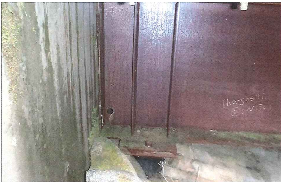
CK2372 Right Abutment bearing
