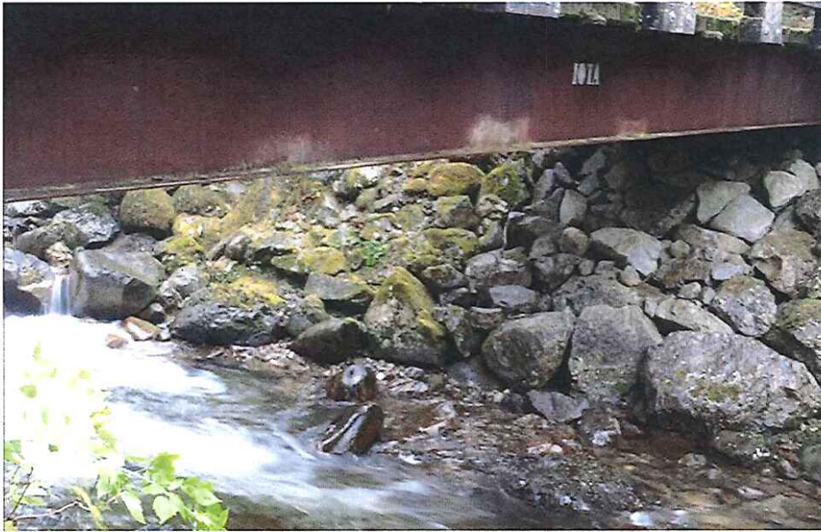
CK2372 From Downstream
