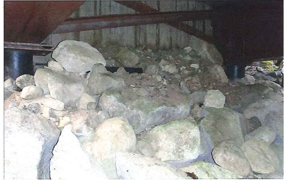
CK2372 Right Abutment
