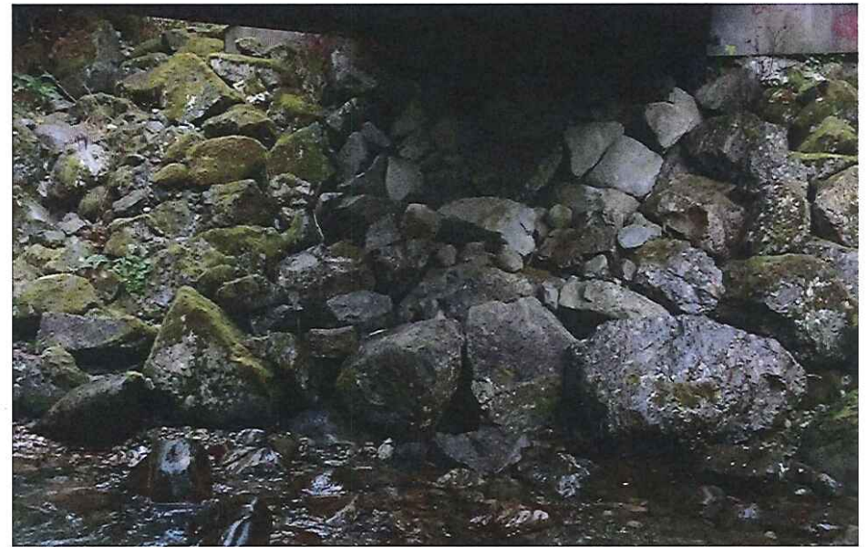
CK2372 Left Abutment
